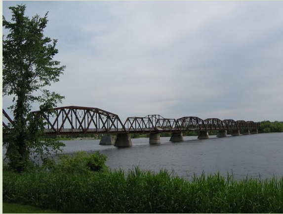
Fredericton former railway bridge
